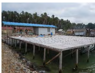
Seaweed drying platform and storage built on the coast (Parang, Sulu)
