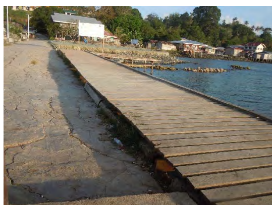
Construction site of fish port complex at Languyan, Tawi-Tawi, by PANAMA program (construction yet to be started)
