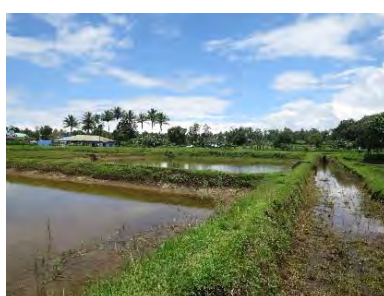
BFAR-ARMM Freshwater fish hatchery at Marantaro, Lanao del Sur. The hatchery facilities are old and outmoded. It produces tilapia and common carp seeds.
