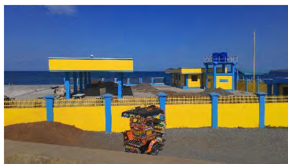
New fishing ports in Lamitan, Basilan, constructed by PFDA Project
