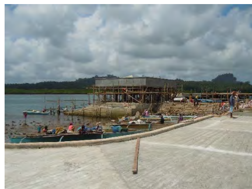
New fishing port in Panglima Sugala, Tawi-Tawi, constructed by PFDA Project
