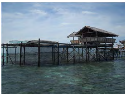
Seaweed drying platform constructed over the water to protect seaweed from sand (Tawi-Tawi)
