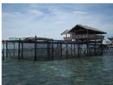
Seaweed drying platforms constructed on the sea to prevent mixing dried seaweed with sands. (Sitangkai, Tawi-Tawi)
