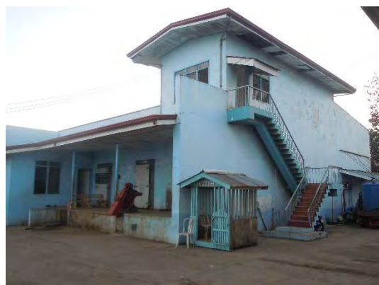
Ice making plant in Joro, Sulu, managed by BFAR-ARMM provincial office
