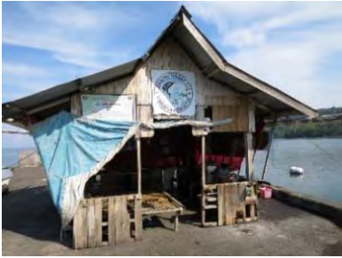
A local office of Bantay Dagat is located on the pier of fishing port at Parang, Maguindanao. It is necessary to renovate the office building.
