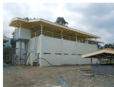
Water reserve tank
