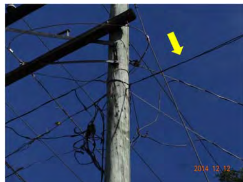
Illegal connection (indicated by arrow)
