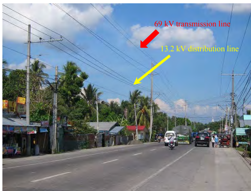
Photo 6.1 Shared Transmission and Distribution Lines in Cotabato City
