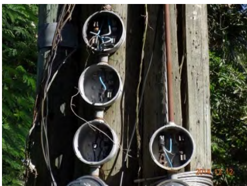
Broken kWh Meter
