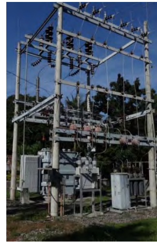
Power transformer without nameplate (year of manufacture, etc. are unknown)
