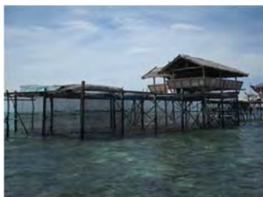
Solar seaweed dryer platforms are constructed on the sea to avoid mixing dried seaweed with sands. (Sitangkai, Tawi-Tawi)
