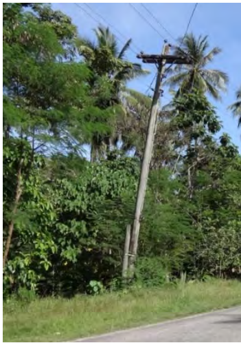
Very old and leaning wooden pole of distribution line with supporting post
