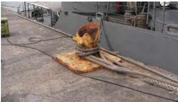
Photo 4.5: Damaged bollard
