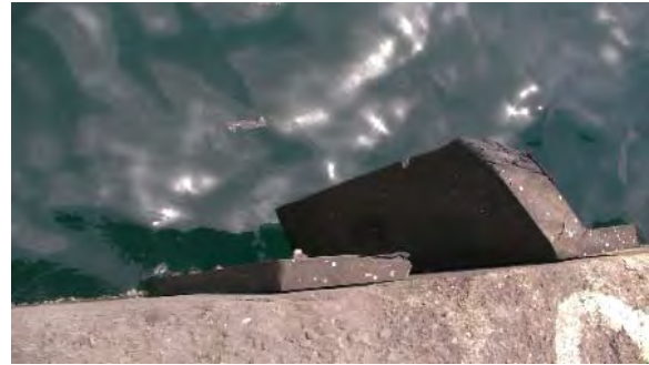
Photo 4.4: Broken fender
