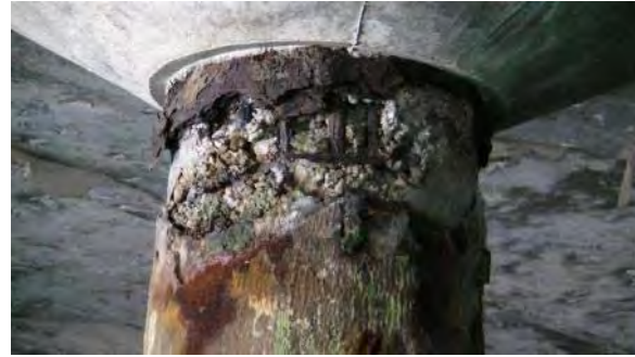
Photo 4.2: Exposed and corroded re-bars
