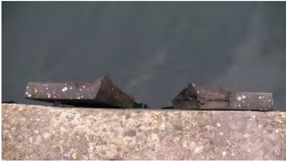
Photo 4.3: Totally damaged fender
