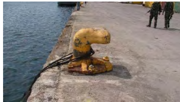
Photo 4.6: New bollard
