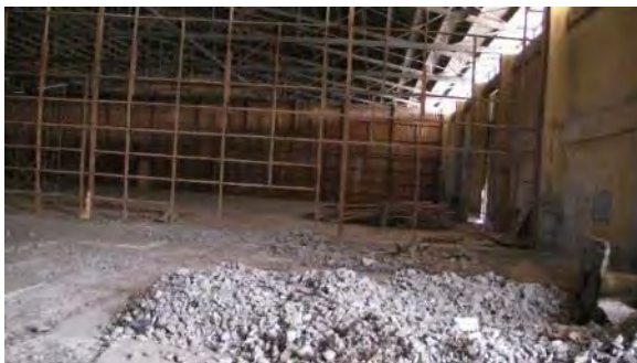
Photo 4.8: Removed concrete surface
