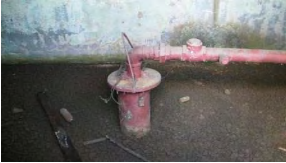
Photo 4.10: Existing deep well
