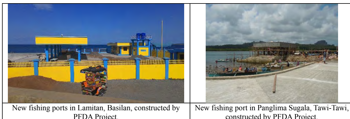
Photo 3.3 Fish Port Complex Construction in PFDA Project
