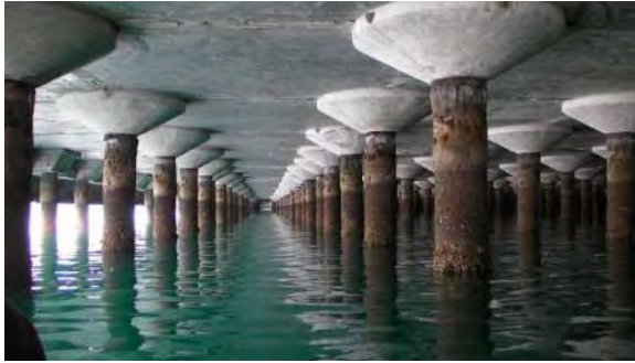
Photo 4.1: Corroded upper portions of piles
