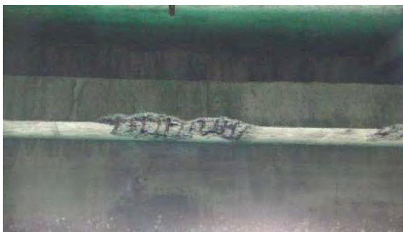
Photo 4.7: Corroded re-bar
