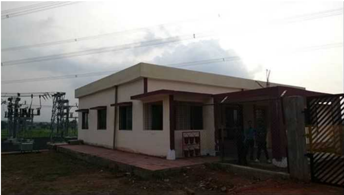
Figure 2-20 Control Building (Tejgarh 132kV Substation)
