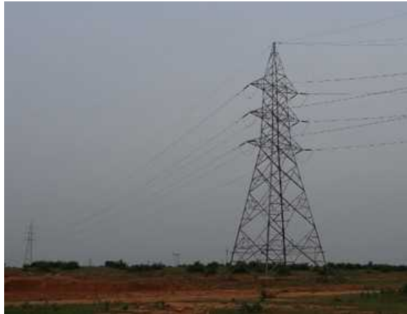
Figure 2-5 (left) 400 kV & (right) 132 kV Transmission Lines
