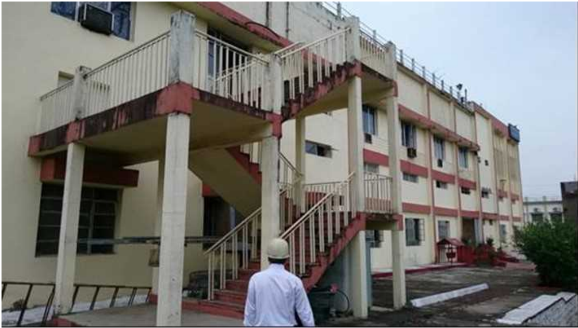
Figure 2-19 Control Building (Jabalpur 220kV Substation)
