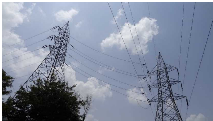
Figure 2-7 LILO System of the 132 kV Transmission Line
