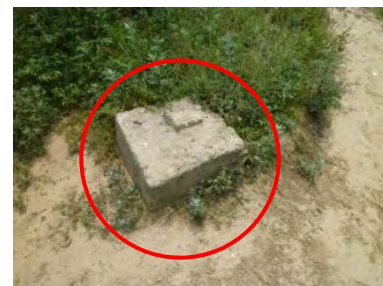
Wasted tower foundation
