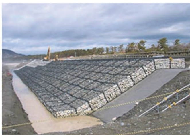
Figure 5-10: A Sample of the Gabion type Revetment in Japan
