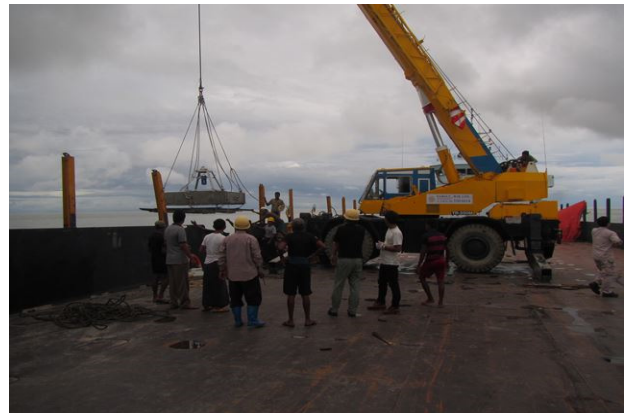
Installation Work of wave Observation on Ship with Crane
