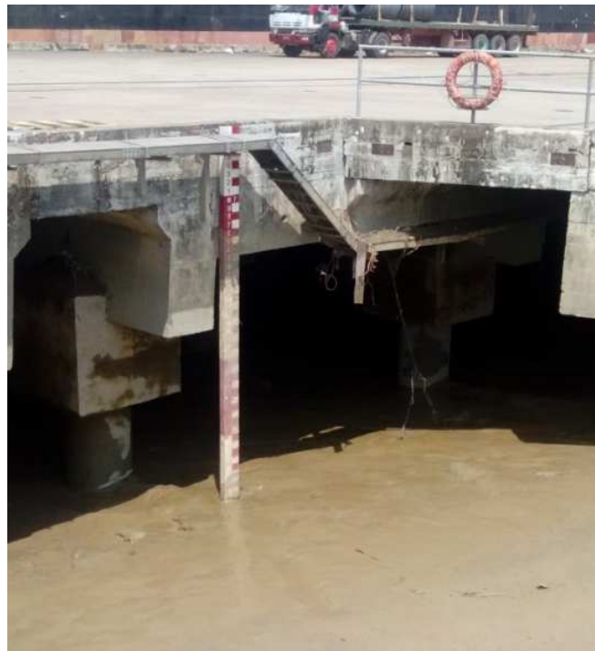
The existing tide staff at Thilawa MITT berth
