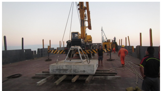
Installation Work of wave Observation on Ship with Crane
