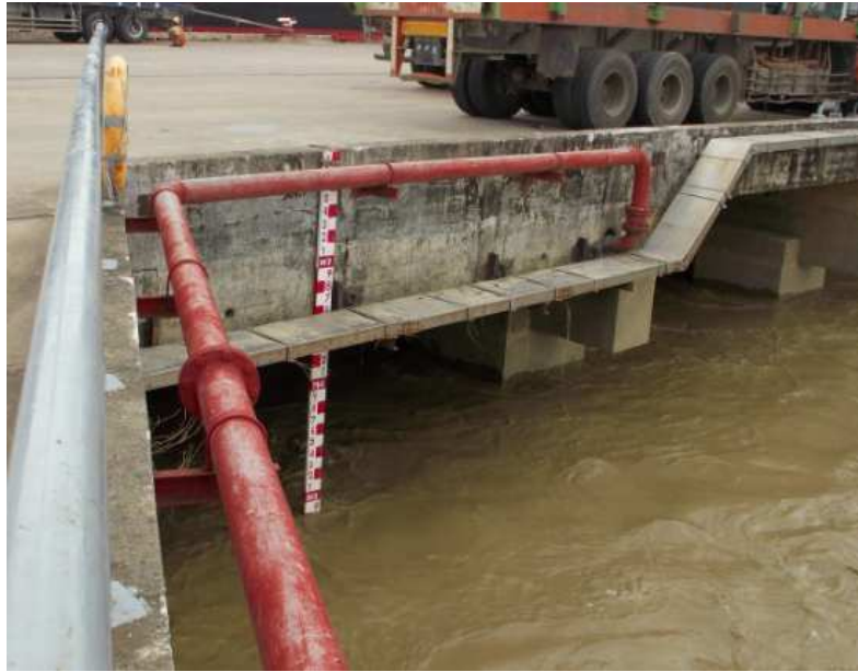
Temporarily established tide staff at Thilawa MITT berth
