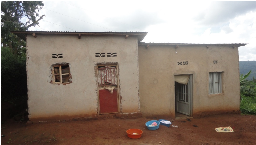
Figure 1-3-2-3.1 Example of Affected Buildings
