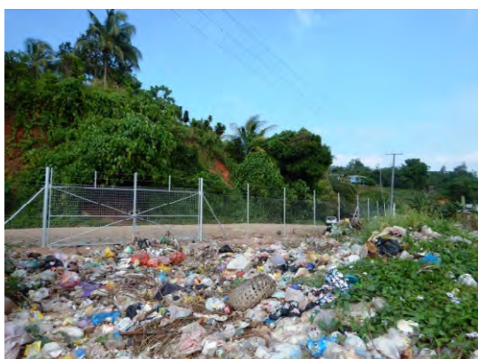
Installation of Fence (August, 2015)
