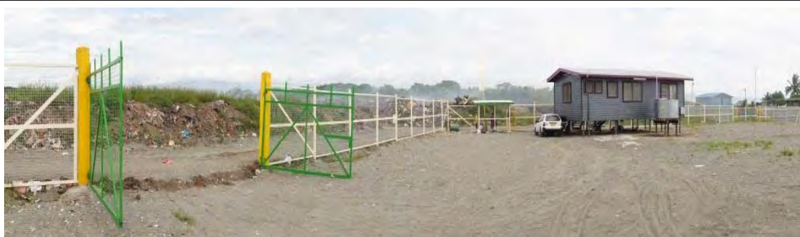
Completion of Administration and Training Center and Fence at Ranadi landfill (May, 2015)
