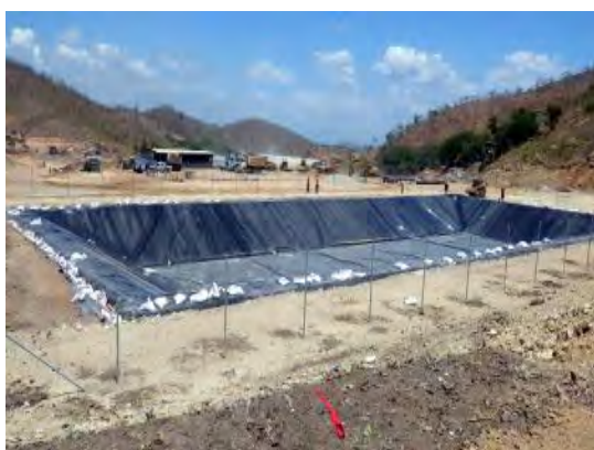
Leachate Treatment Pond, Liner Facility, Fence (December, 2015)
