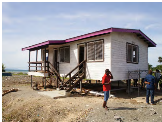
Construction of Administration and Training Center at Ranadi landfill (February, 2015)
