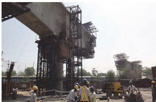
Figure 4.4 An example of the OSV application at Delhi Metro Project
