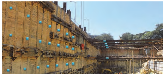
Figure 4.3 A prospect view of maximized OSV monitoring
