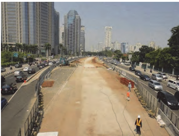
Figure 1.2 Jakarta MRT Construction Site
