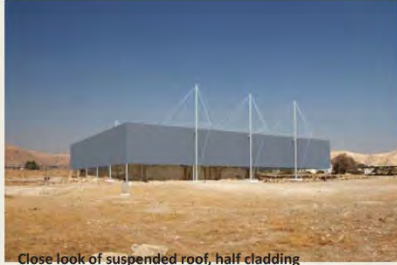
Close look of suspended roof, half cladding
