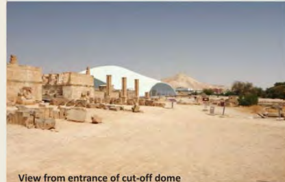
View from entrance of cut-off dome
