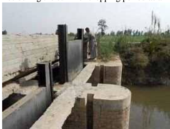
Check Gate on Shaba Canal (KM2.5)
