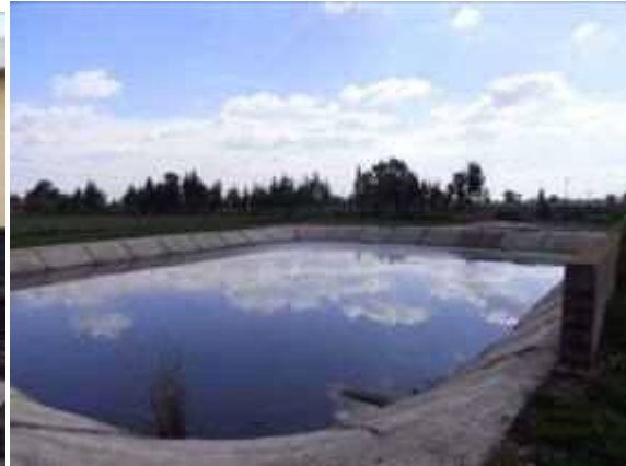
Sedimentation basin in El Mufty village
