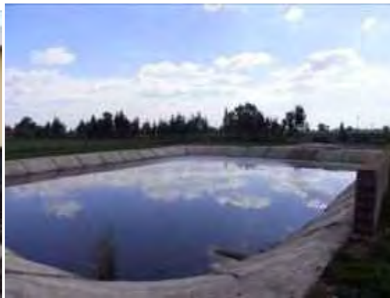
Sedimentation basin in El Mufty village
