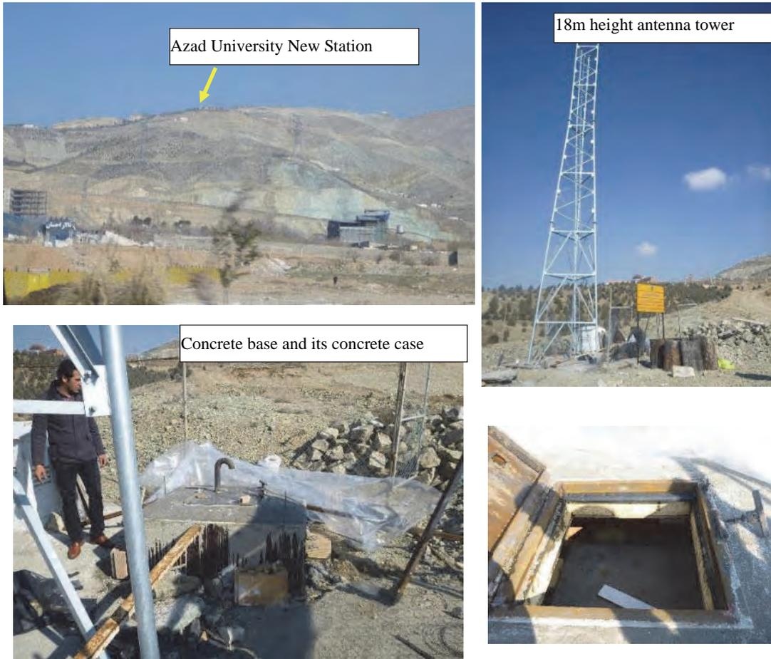
Figure 2.4.5 Construction Works for Azad University Observatory
