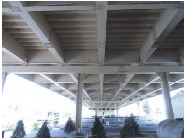
Figure 2.2.26 Photo taken under the target bridge
