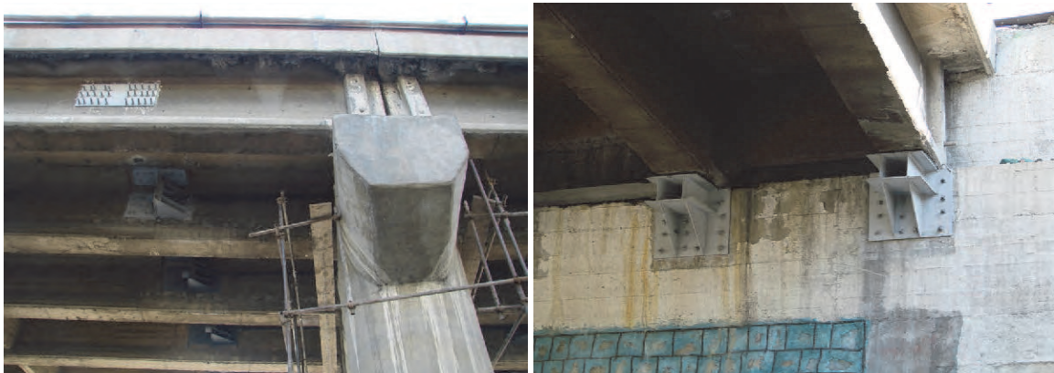
Figure 2.2.29 Photos of Retention device(left) and Bridge seat widening(right)
