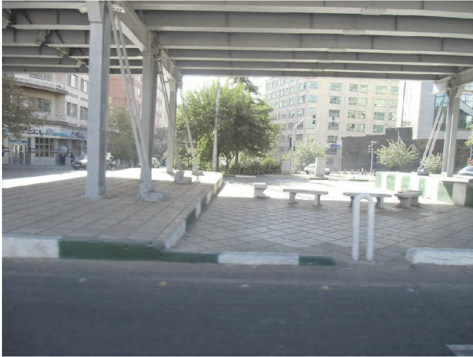
Figure 2.2.28 Photo of bridge with seismic retrofitting implemented
