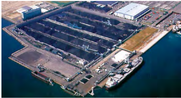
Dust Proofing Fence
