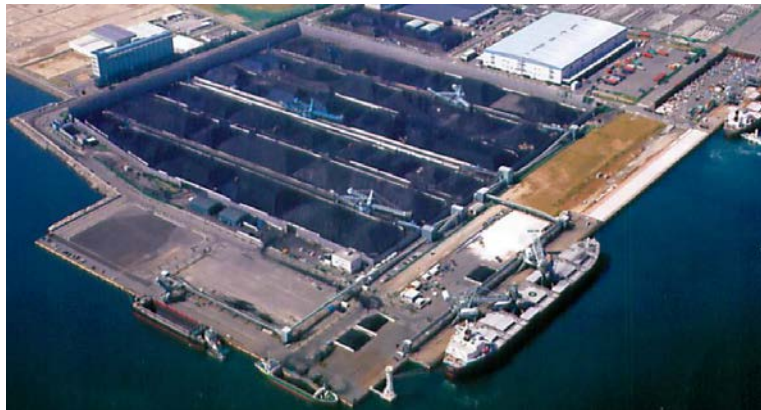
Dust Proofing Fence
