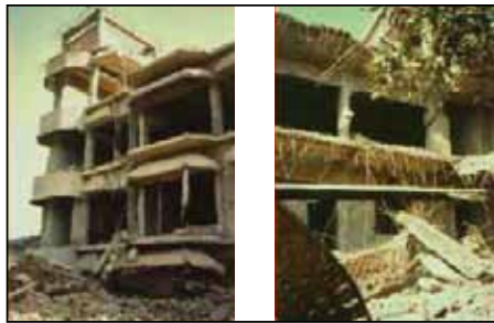
Damage caused by Nov 1997 earthquake in Chittagong
