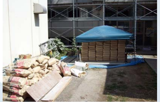
Temporary Shed for stacking cement at field.
