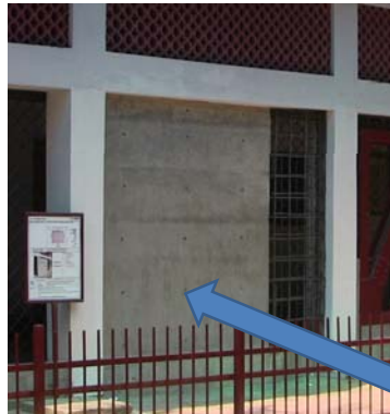
Test Work of CNCRP in 2012
