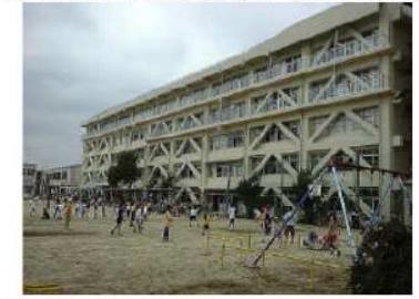
d) Elementary School Building (with Balconies)
