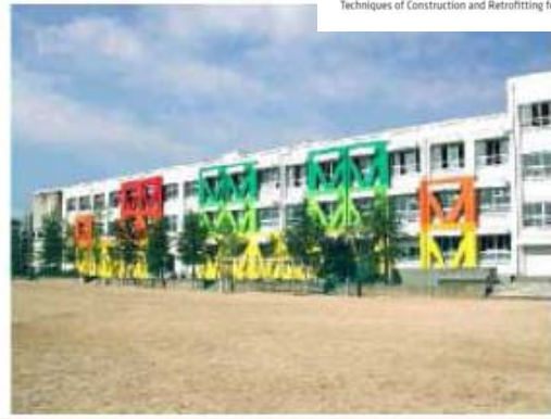
b) Junior High School Building (Designed by Students)
