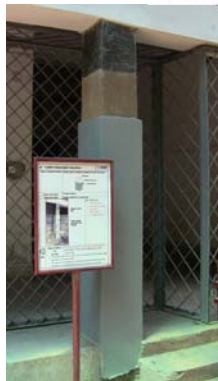
Test Work of CNCRP in 2012
