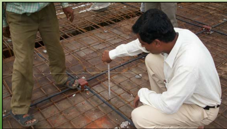
SLAB CHECKING
