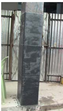
Test Work of CNCRP in 2012
