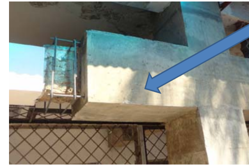
Test Work of CNCRP in 2013
