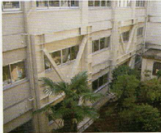
Ookashiwa Elementary School
