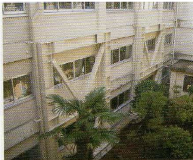
Ookashiwa Elementary School
