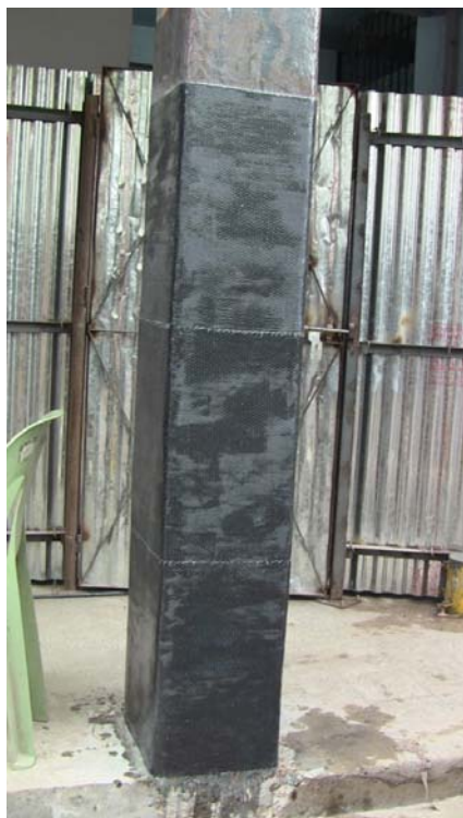
Test Work of CNCRP in 2012
