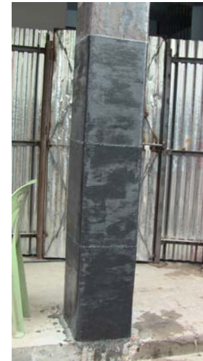
Test Work of CNCRP in 2012
