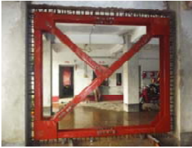
Steel Frame Bracing at Ground Floor
