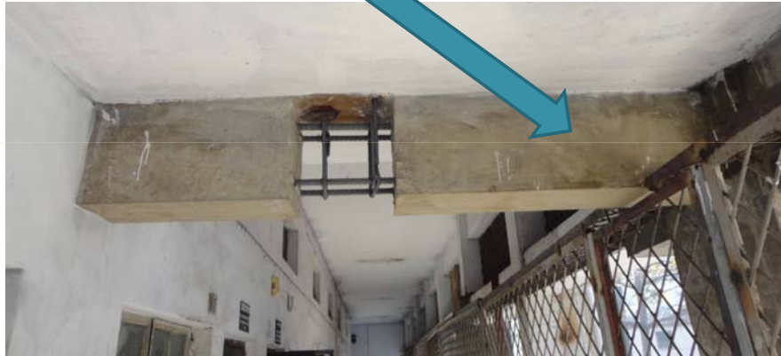
Test Work of CNCRP in 2013
