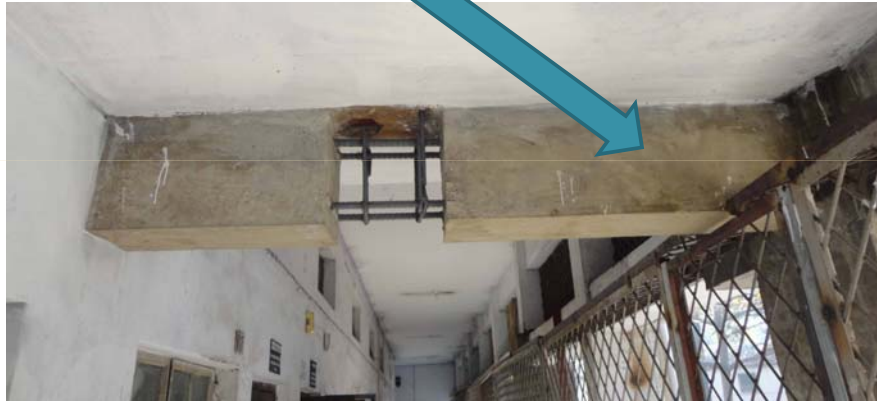
Test Work of CNCRP in 2013
