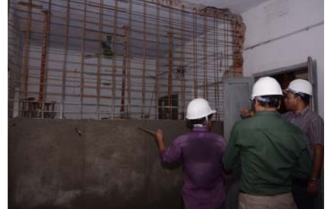
RCC Shear Wall at Ground Floor
