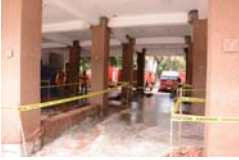
Column Jacketing at Gr. Floor
