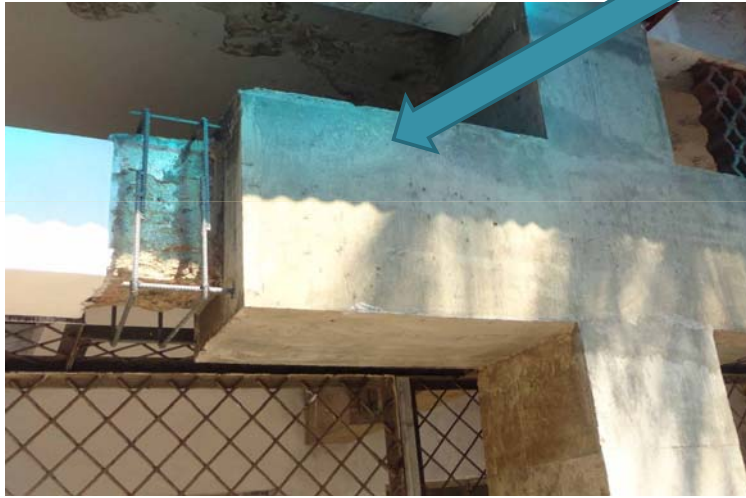
Test Work of CNCRP in 2013
