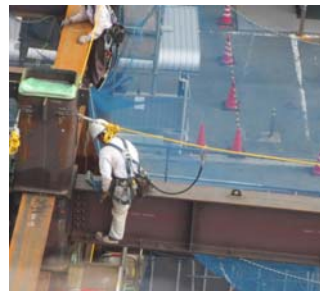
Worker with Safety Harness Site: IDEC Corporation new HQ
