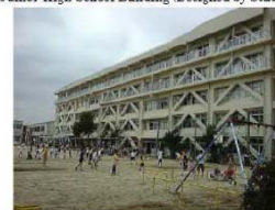
d) Elementary School Building (with Balconies)
