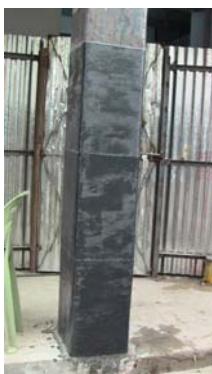
Test Work of CNCRP in 2012
