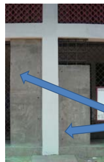
Test Work of CNCRP in 2012
