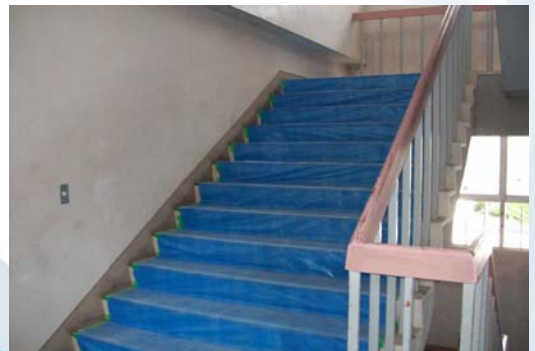
Clean at working site.
