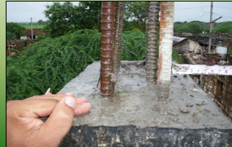
CHECKING OF RCC WORK
