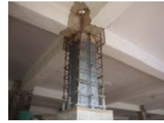
Column Jacketing Work at site
