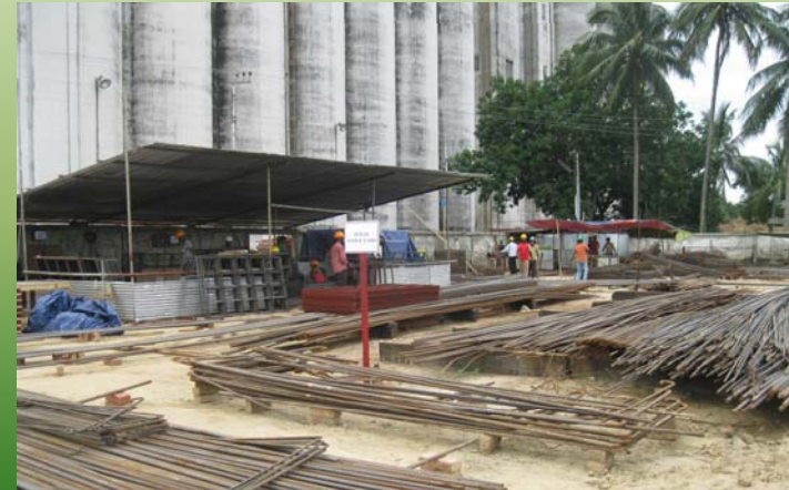
Storage of Rebar
