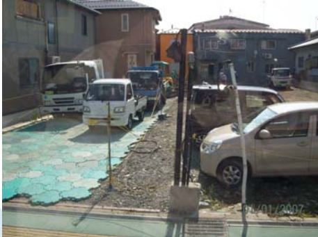
Clean at working site.
