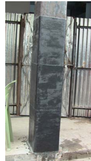
Test Work of CNCRP in 2012
