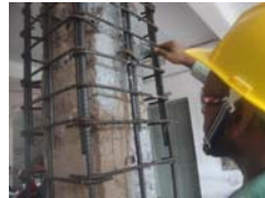
Chemical Applying on old Column Surface
