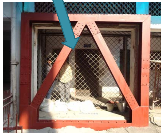
Test Work of CNCRP in 2013
