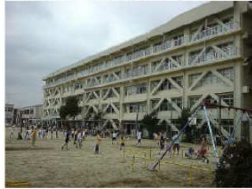
d) Elementary School Building (with Balconies)
