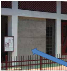
Test Work of CNCRP in 2012
