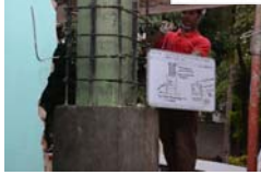
Checking of Reinforcement
