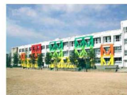
b) Junior High School Building (Designed by Students)
