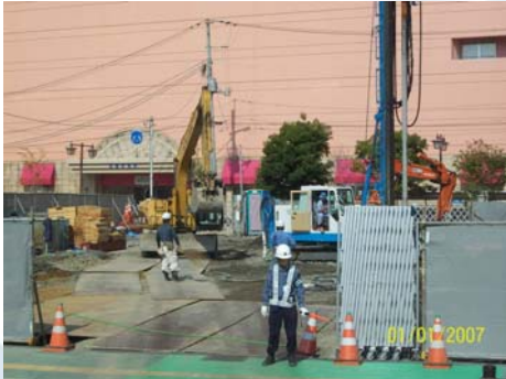
Clean at working site and use of Helmet
