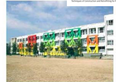
b) Junior High School Building (Designed by Students)
