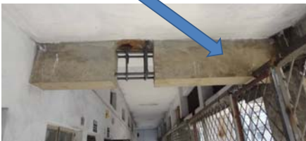
Test Work of CNCRP in 2013
