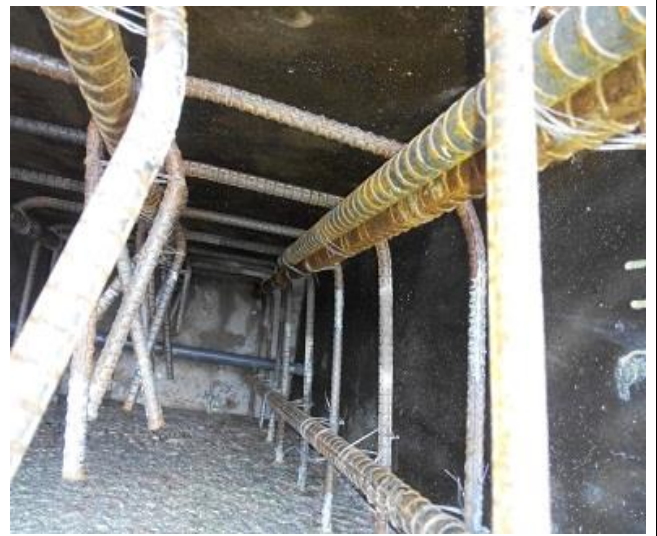
PHOTO 2: Before Casting Shutter inside Condition
