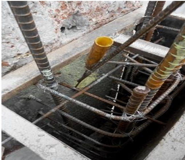
PHOTO 1: Before Casting NETO BOND Applying
