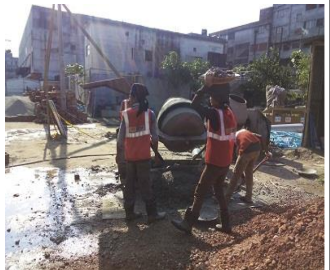
PHOTO 6: Materials Mixing for Concreting Work
