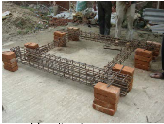
Assembly of re-bar
