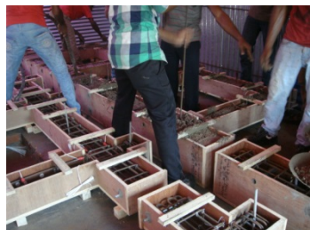
Concreting and surrface finishing
