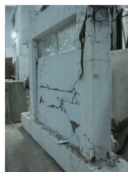
Out of plane movement of brick wall
