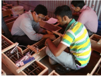
Assembly of re-bar
