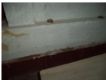
Filler plate at bottom of beam
