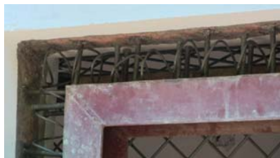
Connection Details, Test Work 2012
