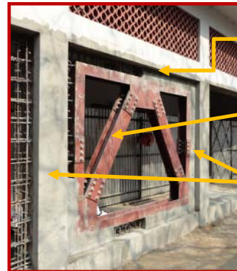
4) Steel bracing
