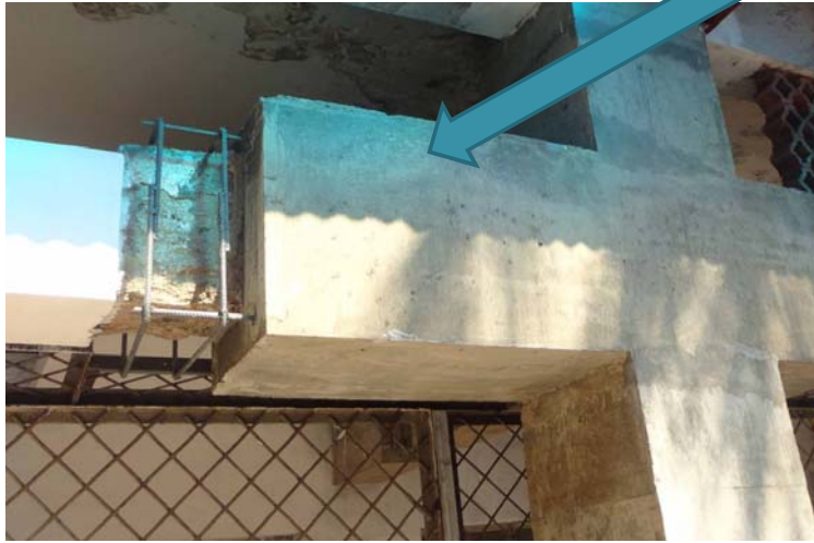
Test Work of CNCRP in 2013
