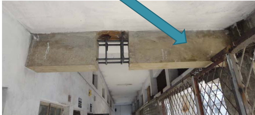
Test Work of CNCRP in 2013
