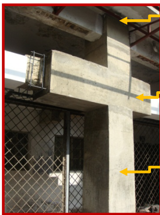
8) Concrete jacketing on existing column
