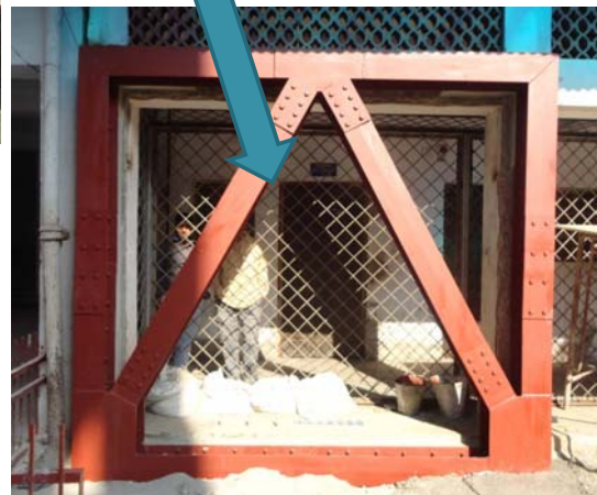
Test Work of CNCRP in 2013
