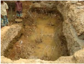
(a) Top of rebar of cast-in-situ piling
