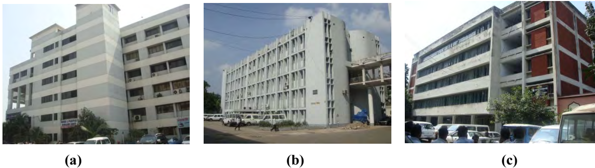
Photo 2.10.1 Candidate buildings for Pilot project
