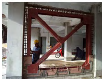
(b), (c) Pressure grouting of non-shrink mortar work
