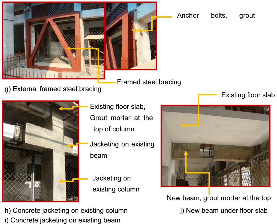
Figure 2.6.3 Construction methods of Test Work (2 nd year)
