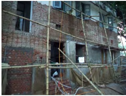
a) Wall re-bar work
