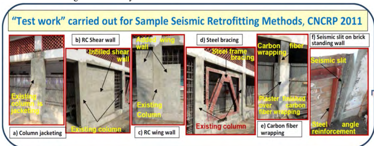
Fig. 7 The Six Types of Retrofitting Construction of the Test Works (2011)
