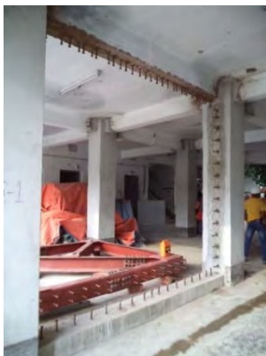
(a) Post installed anchor work
