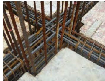
(e) Re-bar arrangement at beam column joint
