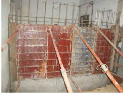
(a) Formwork for RC wall
