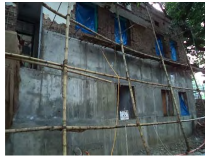
b) Concrete work
