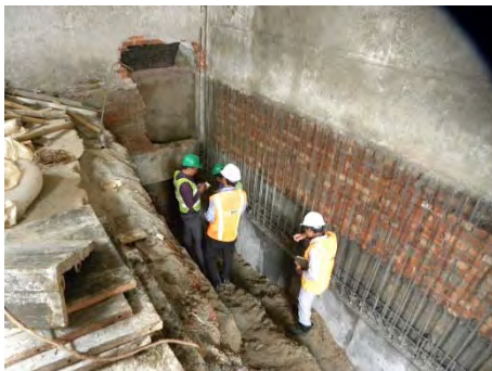
3. Shear Wall Checking
