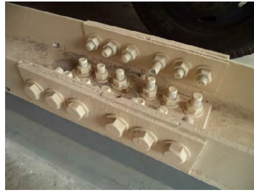
f) Connection of steel member
