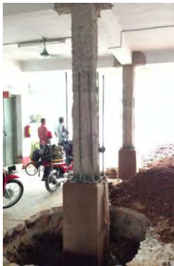
a) Re-bar and concrete work
