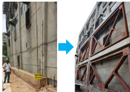
Fig. 15 First Retrofitting Work at RMG Factory by Japanese Loan
