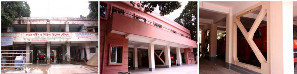
Fig. 11 Pilot Project (left: before, center: after retrofitting, and right: steel bracing)
