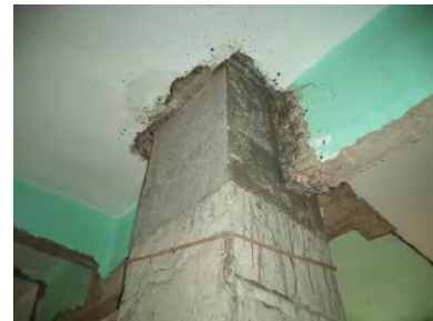
c) Non-shrink mortar pressure grout work
