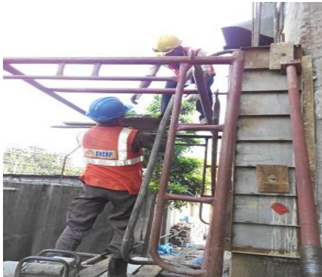
PHOTO 3: Casting Materials Taking for Placing
