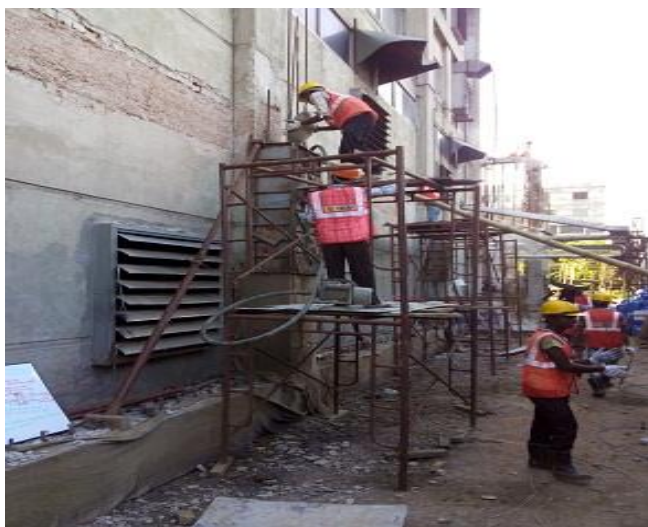
PHOTO 5: Concreting Works Going On
