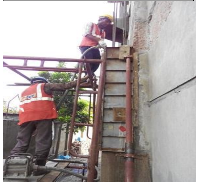
PHOTO 4: Vibrator Applying into Casting
