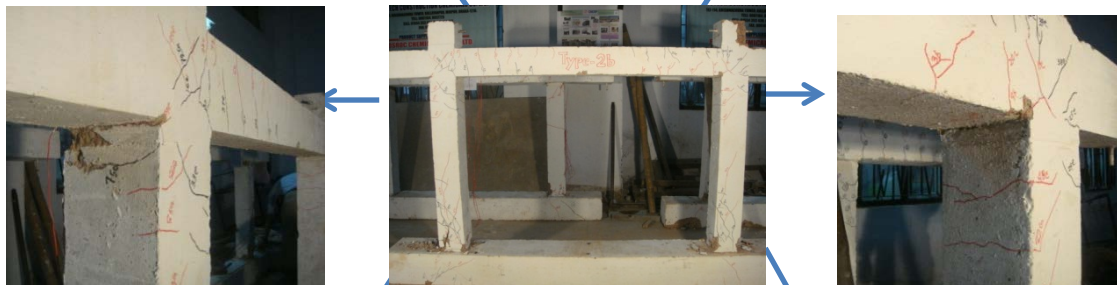
Compressive failure of covering concrete
