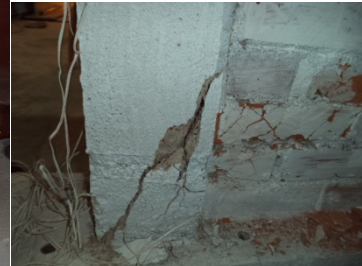
Shear failure of right column (front and rear side)
