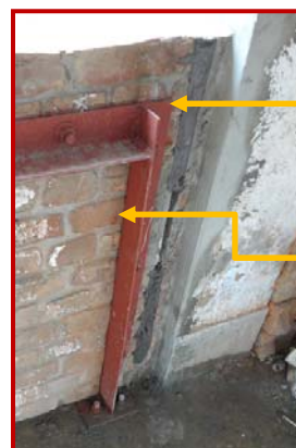
6) Seismic slit on brick standing wall
