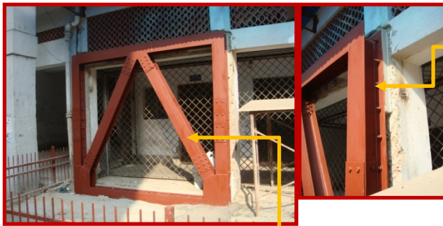
7) External framed steel bracing
