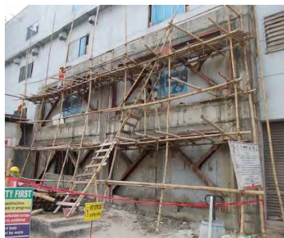
4. Steel Frame Bracing
