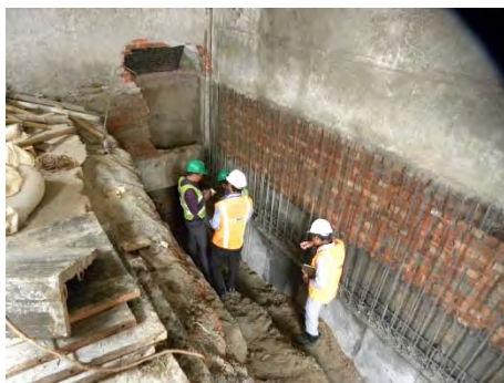
3. Shear Wall Checking
