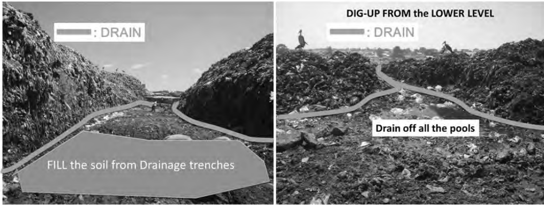
Figure 5: Drain 2 Drain on Both Edges (combination of rainwater and leachate)
