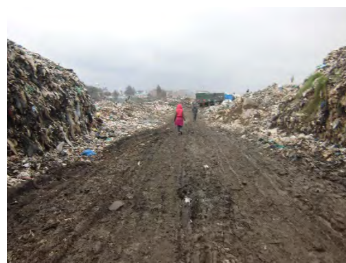
Photo 2-3 Road Improved by Compaction with Hard Core
