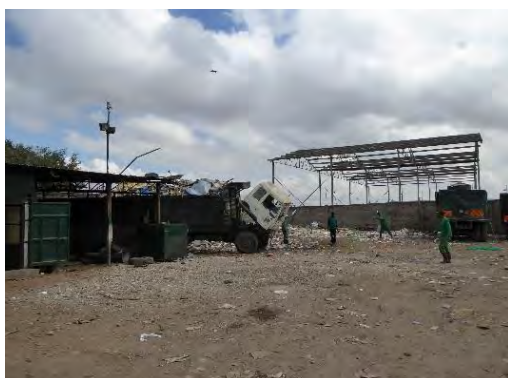
Photo 2-30 Waste Transfer Facility
