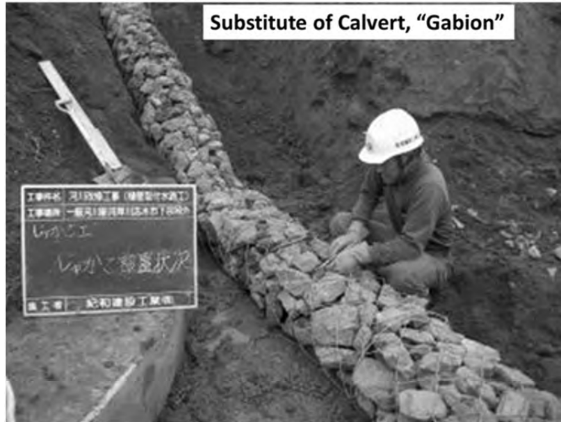
Figure 8: Installation of Gabion (substitute of culvert)
