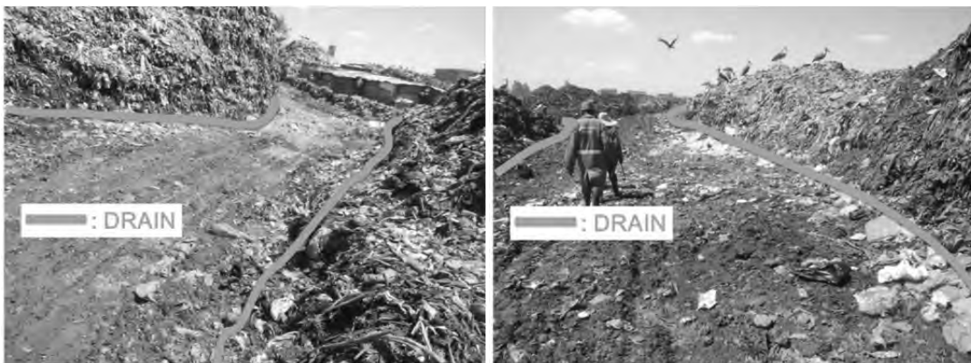
Figure 4: Drain 1 Drain on Both Edges (combination of rainwater and leachate)
