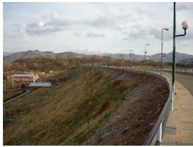
Dam Body of Mahabad Dam
