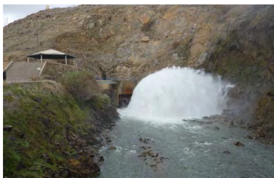
Release of Environmental Flow (about 3\text{m}^3/\text{s} ) from Bukan Dam
