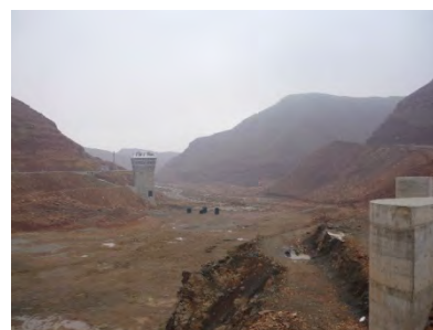
Reservoir Area and Intake Tower (Left Side) of Shahid Madani Dam
