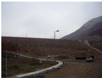
Dam Body of Shahid Madani Dam
