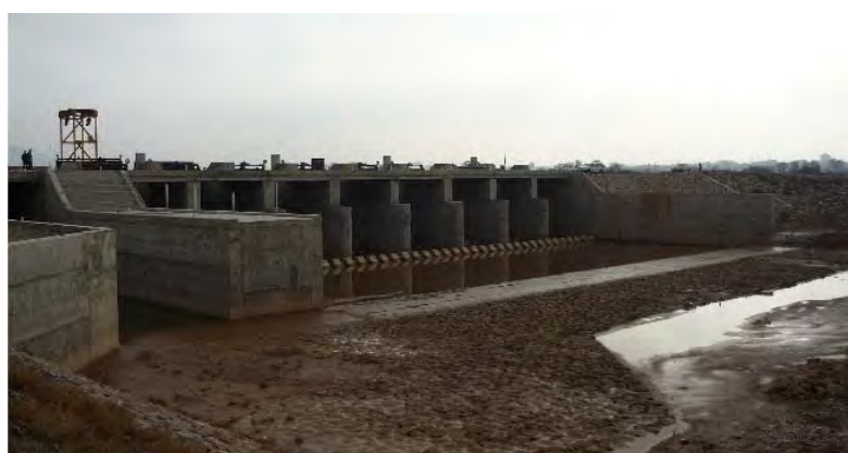
Figure 3.2.5 Relatively Old Intake Weirs for Agriculture and Irrigation Canal in the Aji Chay River
