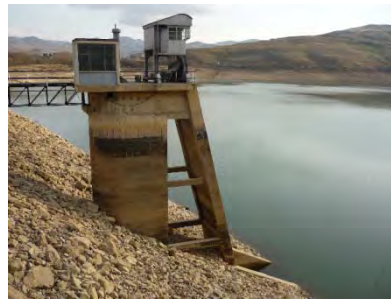
Reservoir and Intake Tower of Mahabad Dam
