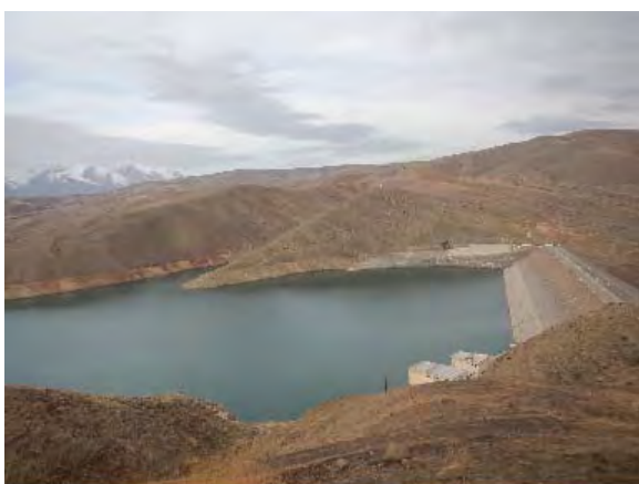
Dam Body and Reservoir of Sharchay Dam
