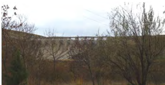
Dam Body of Bukan Dam
