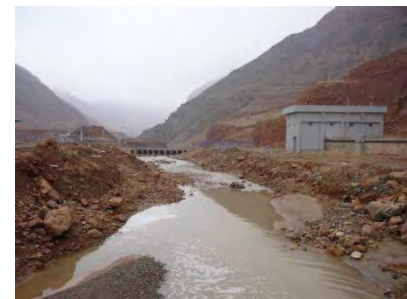
Downstream View from Shahid Madani Dam
