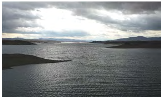
Reservoir of Bukan Dam
