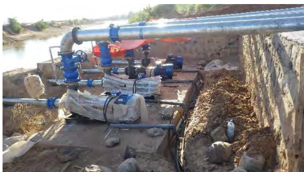
Electric arrangement for motor & pumps had been done (left photo), and test run was started lifting the water to the discharge sump.
