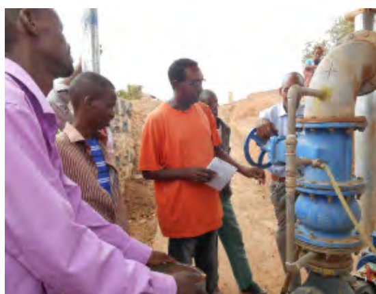
Training on pump facilities and operation (Badilaid)
