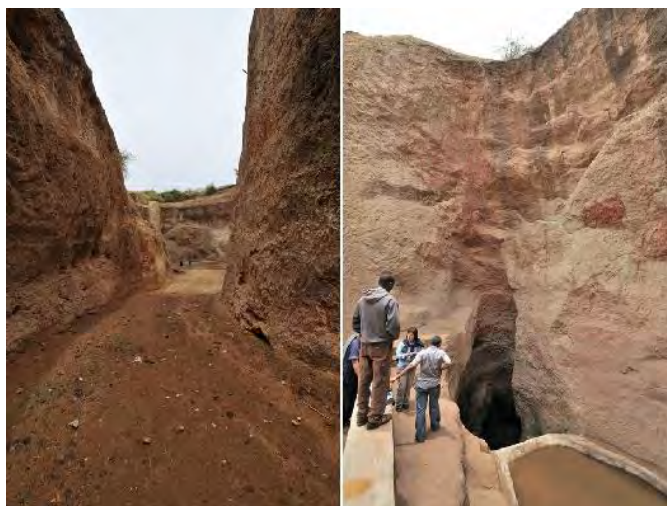
A typical ella found in Dire woreda (right photo). Left photo shows the trench leading to the water point through which cattle are brought down for watering.
