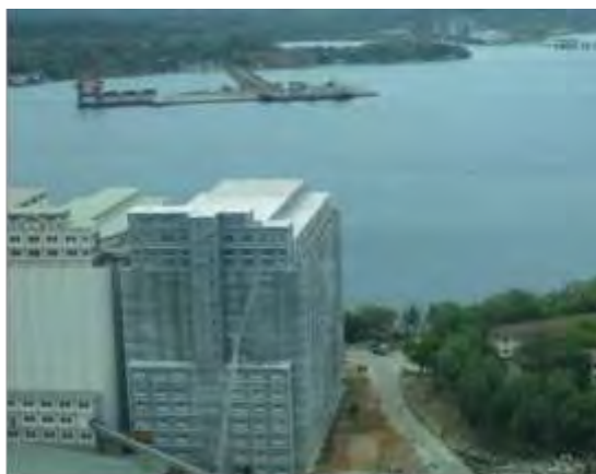
Figure 6.42 Trincomalee cargo berth behind the Tokyo Cement Factory
