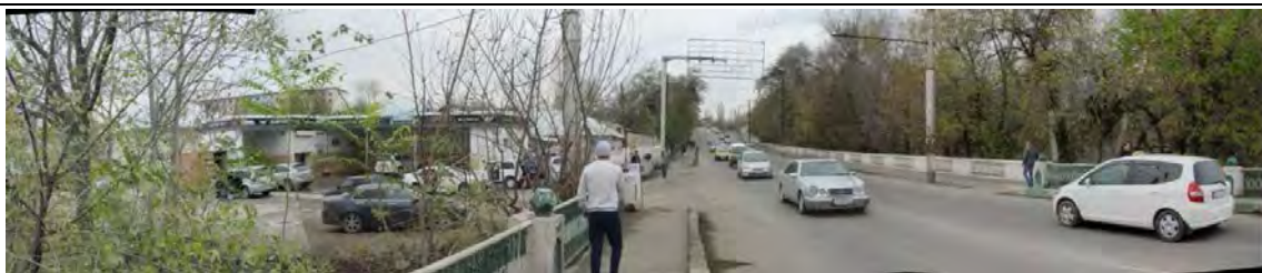
3. The west end of the bridge looking to the western T-intersection
