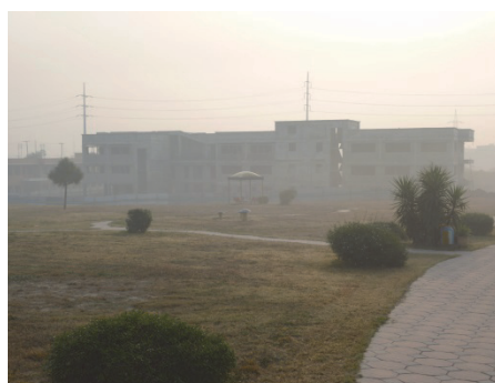
Photo 1: Construction of the ICT Center
