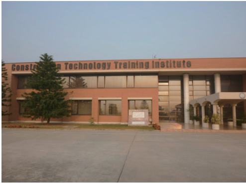
Facade of Construction Technology Training Institute (CTTI)
