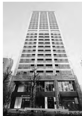
Effective use of space by moving substation underground
