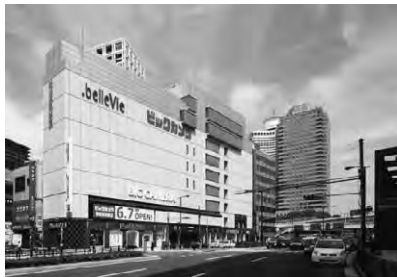
Effective use of available land above a station
