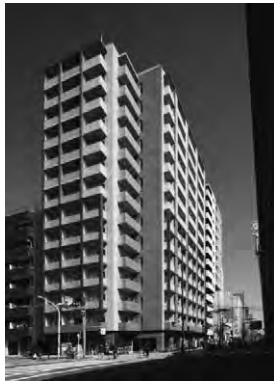
Effective use of land that had once been used for storing materials during construction
