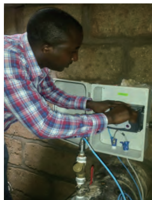
Photo 2. A former trainee is installing equipment for non-revenue water measurement.
