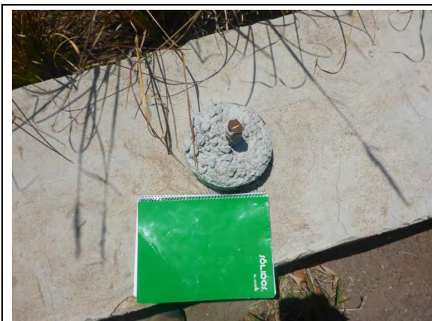
Foto N1.5: Micro pilas \phi = 20\text{cm} (Mar.16, 2015)
