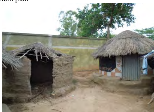
Photo 2 (Two huts subject to demolition)
