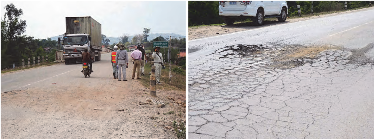
Figure 1.4.11 Damaged Access Road Surface at Xe Tha Mouak Bridge
