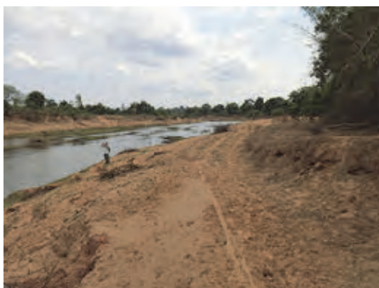
Figure 1.2.34 River bank on the downstream side
