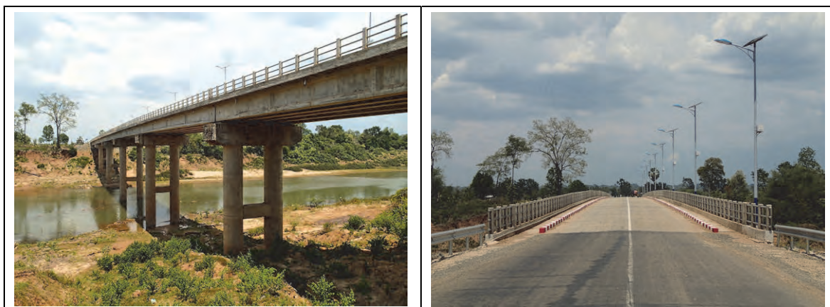
Figure 2.2.7 Bridge Techniques by Lao's Contractor (Sedong Bridge on 15A)
