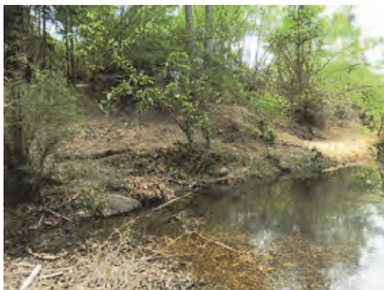
Figure 1.2.32 Riverbank on the upstream side
