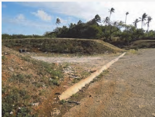
A small ditch for drainage of rain water, developed by MoH C/P (Sep. 2014)
