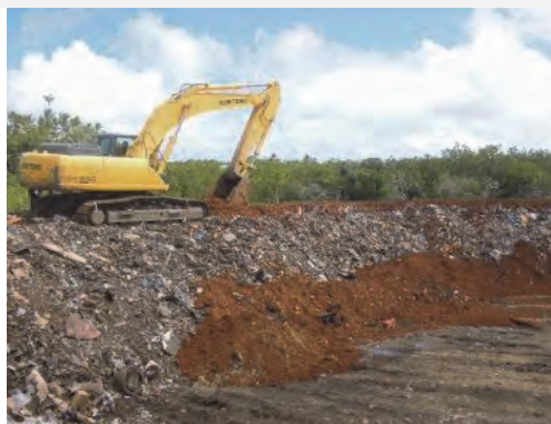
Soil covering at Kalaka landfill (Nov. 2015)
