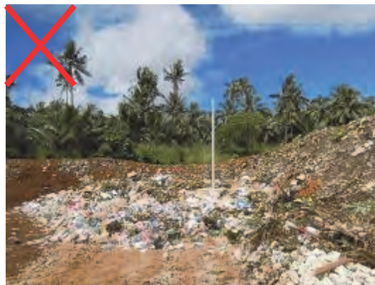
Waste disposed on the access road (Need to avoid being this situation!)
