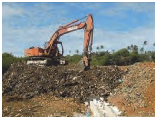
Compacting waste and creating side slope
