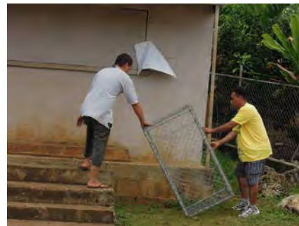
Installation of cages by VEVE Committee (Tu’anequivale)
