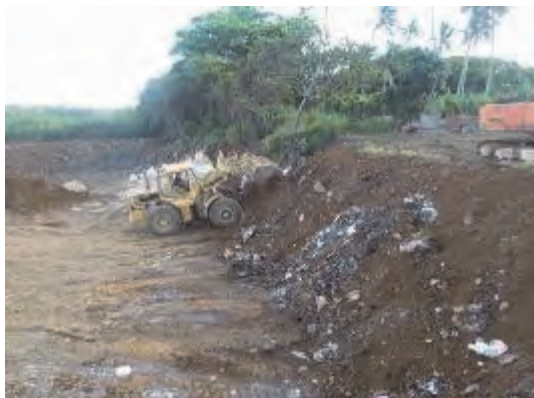
Pushing of waste and soil covering by loader
