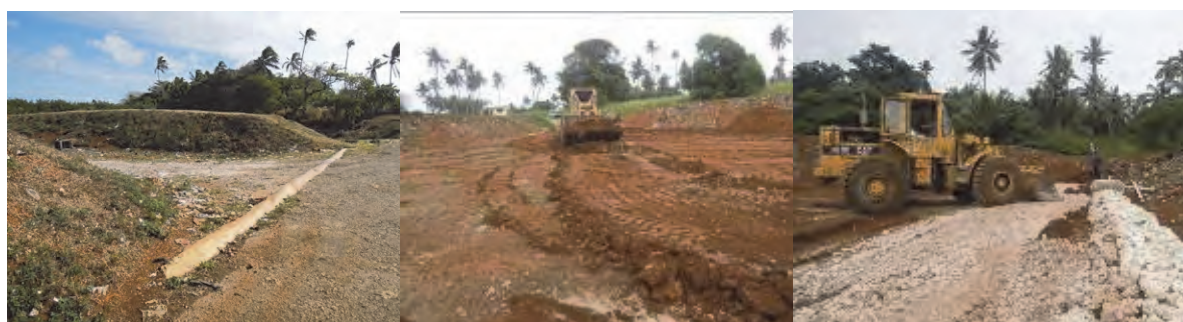
Heap for drainage of rain water
