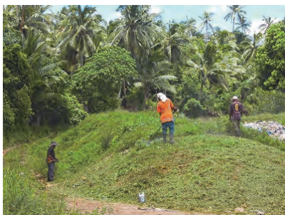
Cutting grass on the embankment
