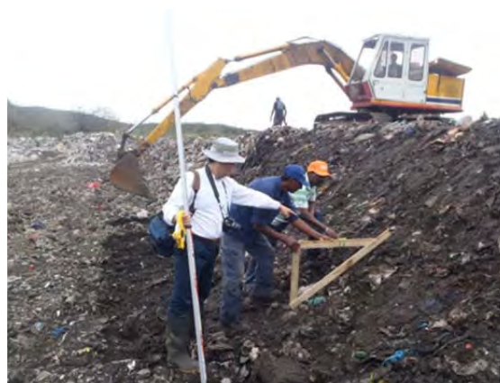
(b) Checking slope gradient (1:1.5)
