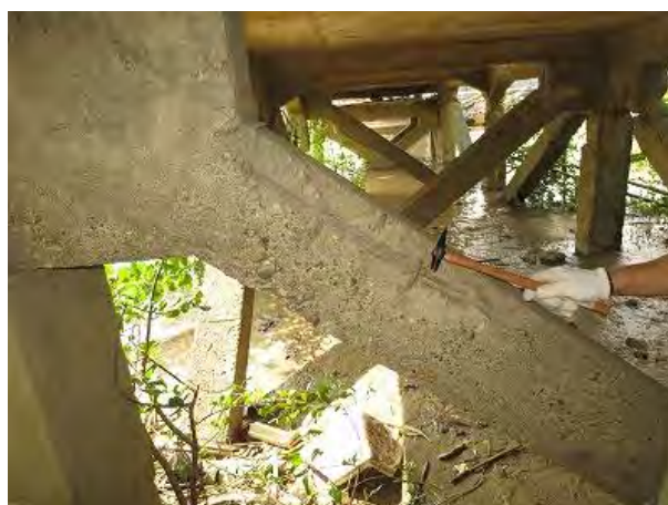
Photo 3.14 Overall and Deteriorated Part (Rebar Exposure) of Wadan Jetty 6
