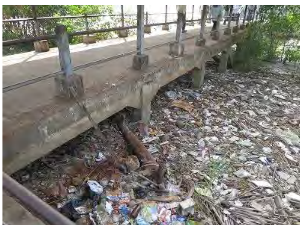
Photo 3.14 Overall and Deteriorated Part (Rebar Exposure) of Wadan Jetty 6
