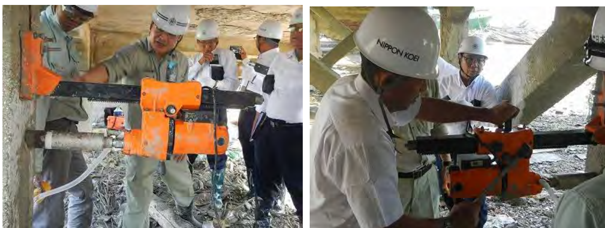
Photo 3.18 Demonstration of Core Drilling and Participant's Operation
