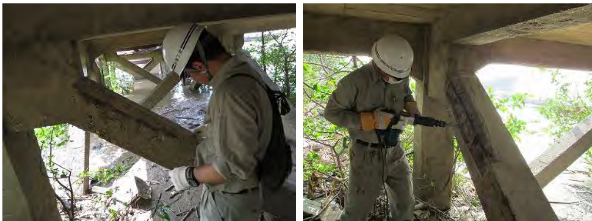
Photo 3.21 Condition of Deteriorated Jetty and Demonstration of Chipping
