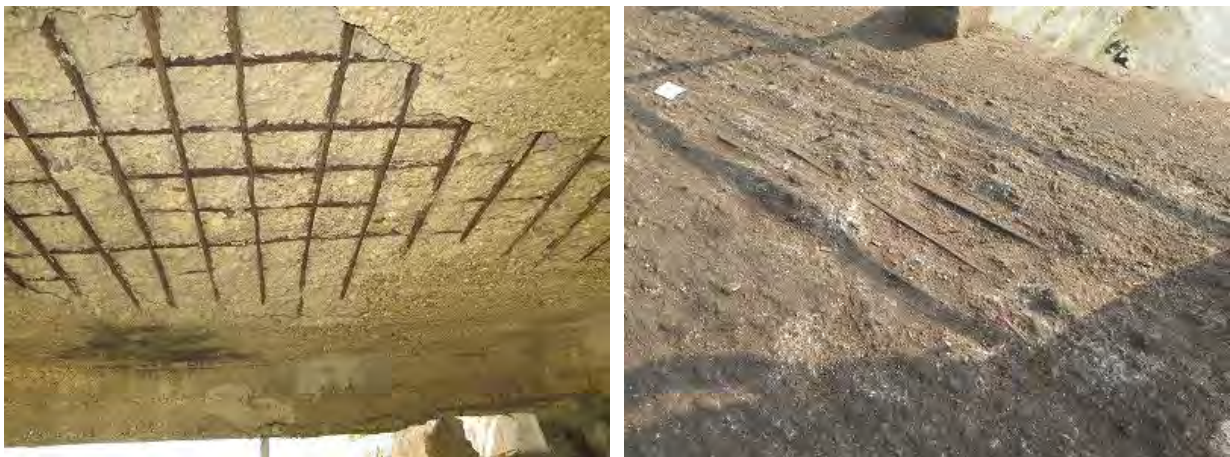
Photo 3.6 Damaged Part on Sin Oh Dang 1
