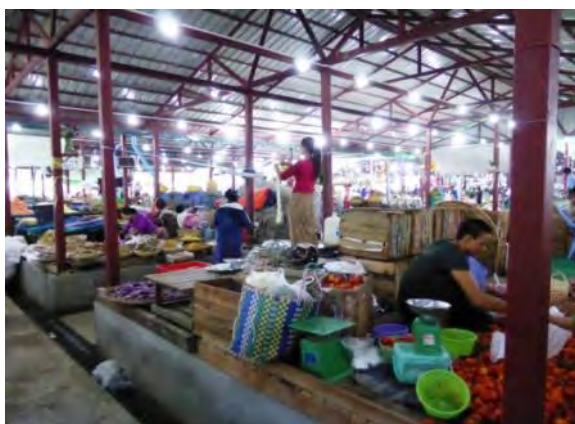
Sanitary condition is secured in 41 Street Zay market. The floor is raised by 50cm concrete base.
