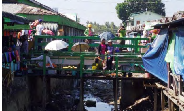
Drainage running along almost center of the Pathein market, giving unsanitary environment to the market
