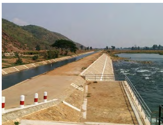
Photo shows the Left Main Canal of Paunglaung irrigation system (right is Paunglaung river) Hydraulic structures in mid-lower parts of the canals have not yet been completed.
