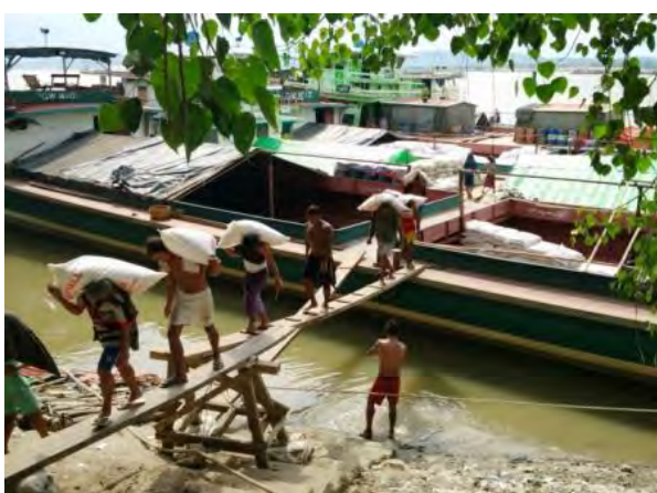
Most parts of berth are natural river bank, and narrow wooden board is used for loading/unloading of cargoes and passengers.
