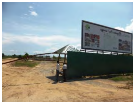
Place where new Mandalay wholesale market is to be established, in a total 205 acres lot.
