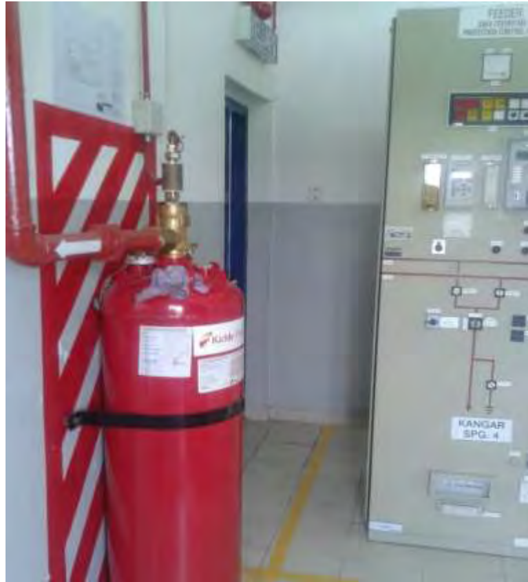
Figure 5: The wall needs to be extended for additional control panel
