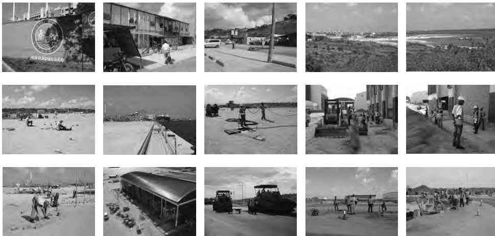
Mombasa Port Development Project - Site Photos (09/Oct/15) (1 of 3)
