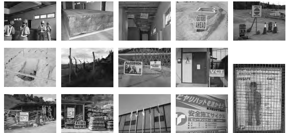
Mombasa Port Development Project - Site Photos (09/Oct/15) (3 of 3)
