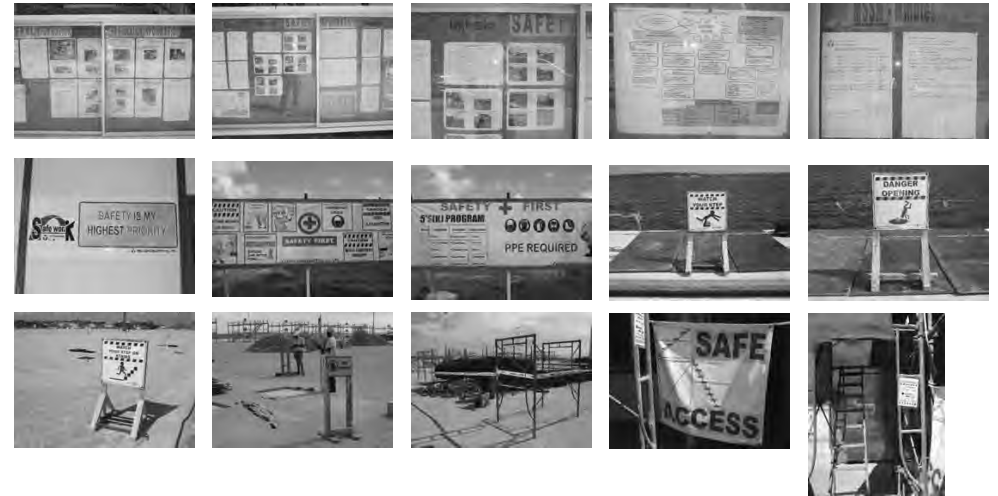
Mombasa Port Development Project - Site Photos (09/Oct/15) (2 of 3)
