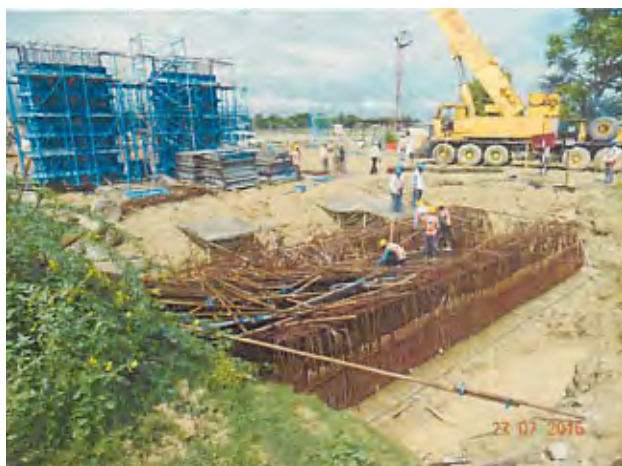
Figure 4.3.11 Vertical Steel for Viaduct Pier Collapsed Due to Failed Support
