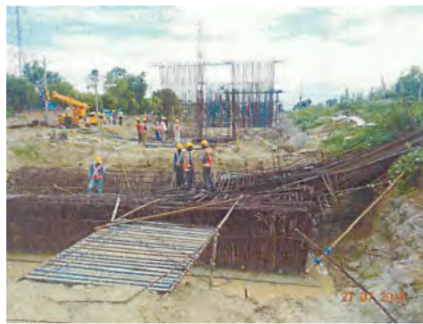
Figure 4.3.11 Vertical Steel for Viaduct Pier Collapsed Due to Failed Support
