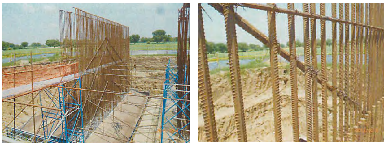
Figure 4.3.2 Situation after Countermeasures Were Applied
