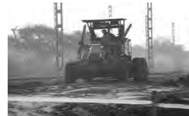
Grader working under supervision
