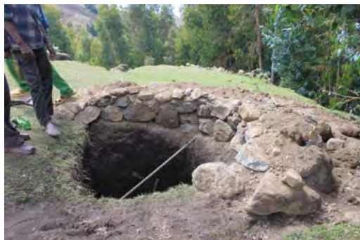
Building toilet at Argin
