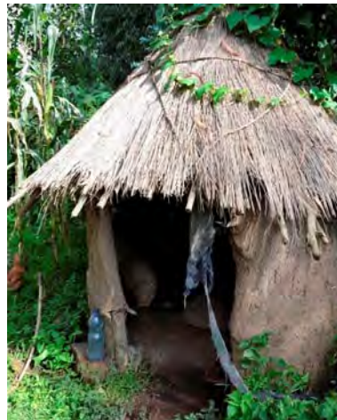
Toilet at Dib Bahir
